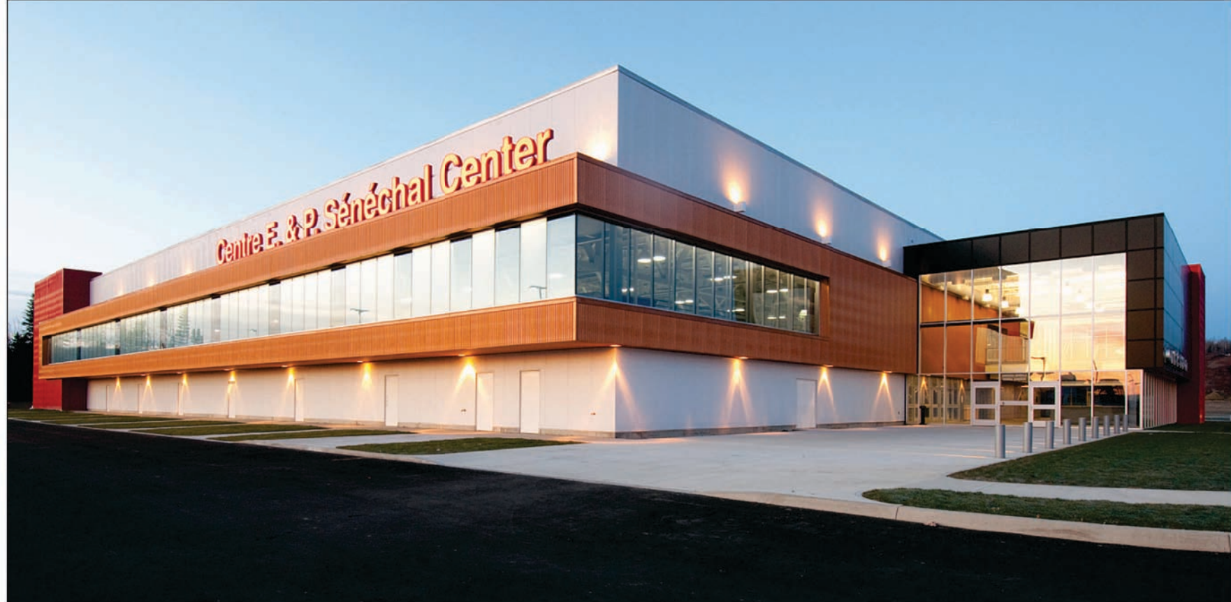
Natural light The walking track extends outside the E & P Sénéchal Centre's exterior walls, using natural light to help increase energy efficiency in the building. Murdock & Boyd Architects Inc. of Saint John won a design award for the building's design last week. (Contributed photo)
